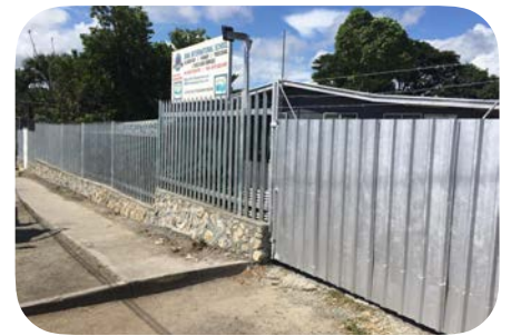
Carpark/walkway repaired by our own efforts
